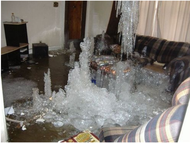
Frozen water pipe damage (© 2015 Showing Suite Inc.)
